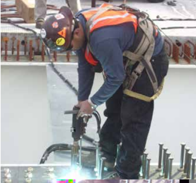
▲ It is important to take into account the nominal melt-off length to determine the required stud length for the application.
