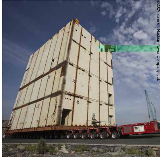
▲ An SC module being transported at a job site.
