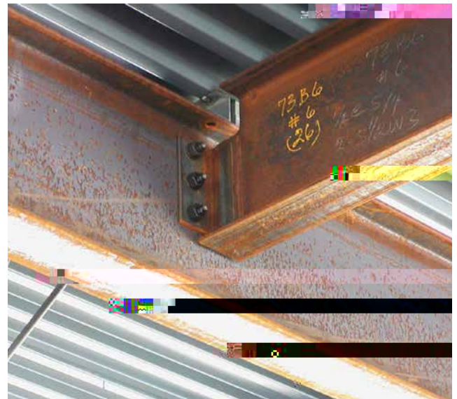
▲ Figure 1. Beam coped at the top flange.
